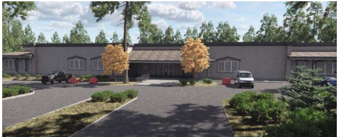
Building being renovated at 125 Crown Point Court in Grass Valley
